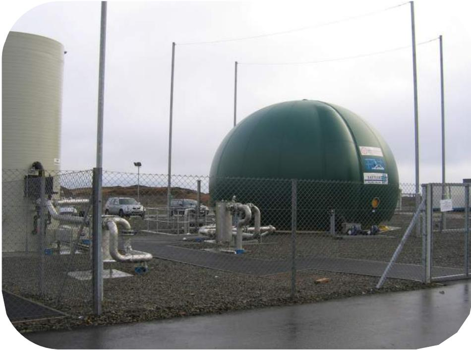
ENER-G has designed, built and delivered a 305 kWe biogas CHP unit for this site, which enables the biogas produced from the AD process to be used to generate enough electrical power to power the site with the surplus being exported to the local network.
